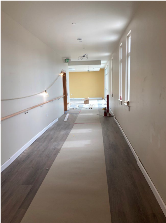
Corridor flooring and handrails installed.
