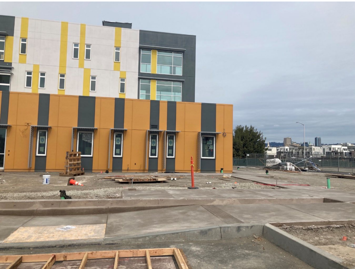
Courtyard cement forms and pours completed.
