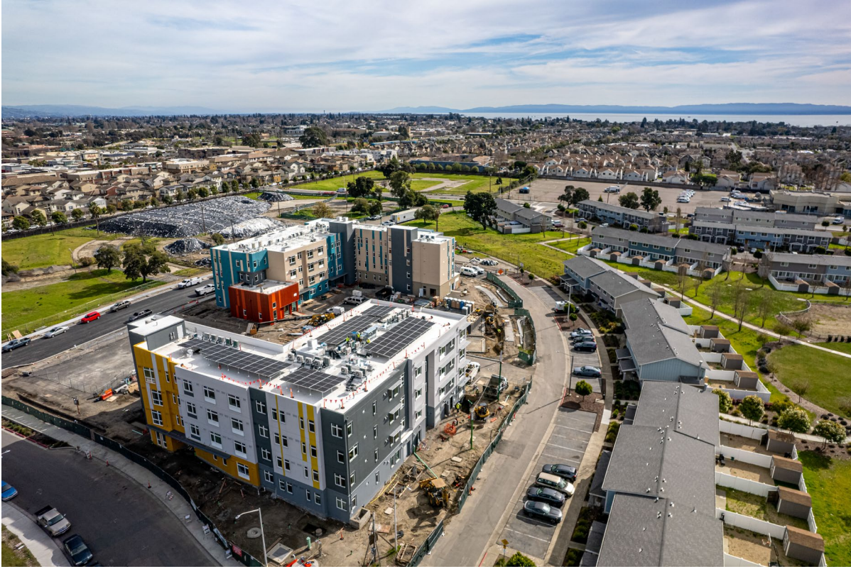
Aerial photo looking south showing the northern and western elevation exterior walls.
