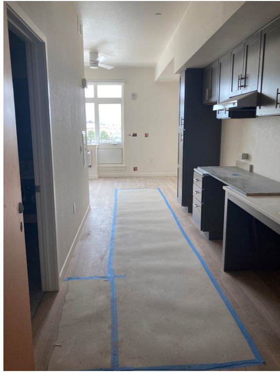
Unit Blinds and Flooring installed.
