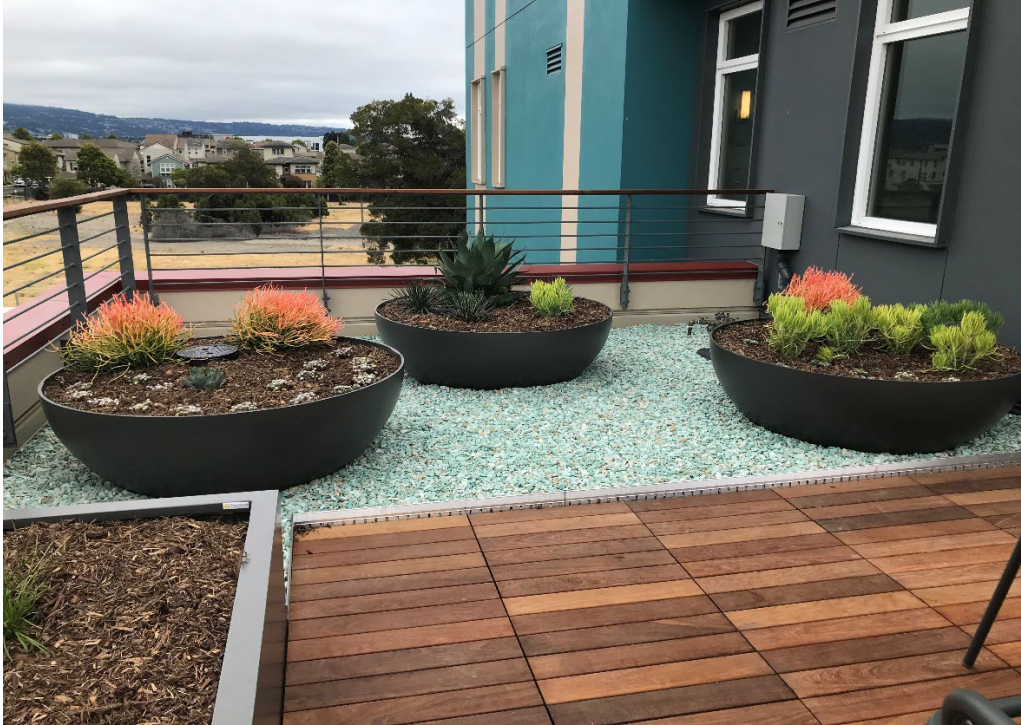
Figure 7: Planters and wood pedestal pavers on third floor roof terrace
