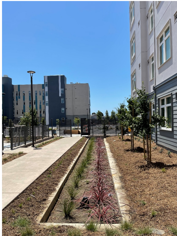
Southern side of Estuary I Landscaping and bioretention area complete
