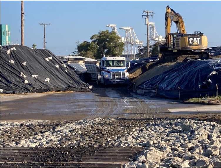
A truck loaded for off haul delivery from excavator.
