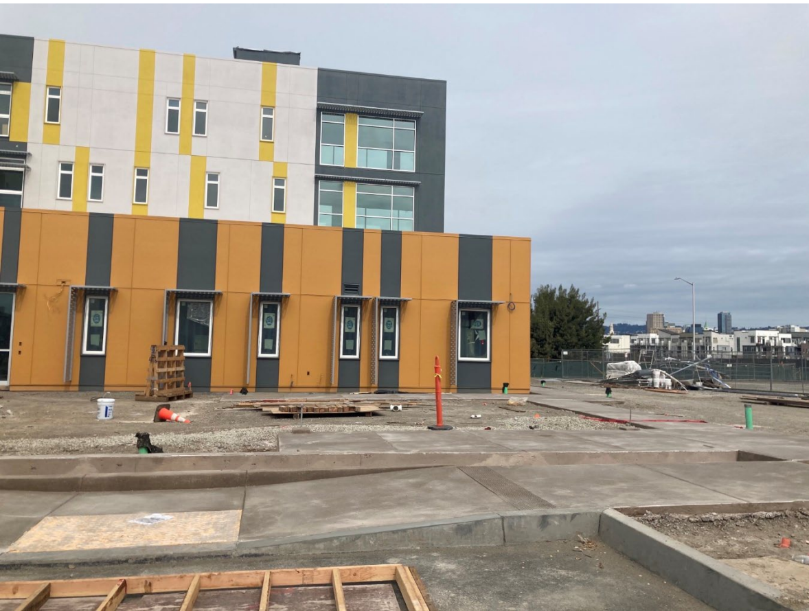
Courtyard cement forms and pours completed.
