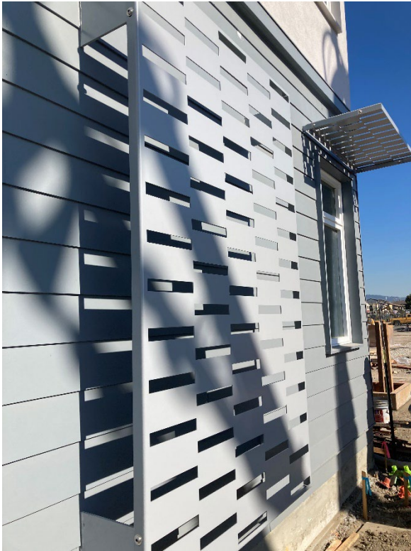
Metal sunshades are installed at the building
