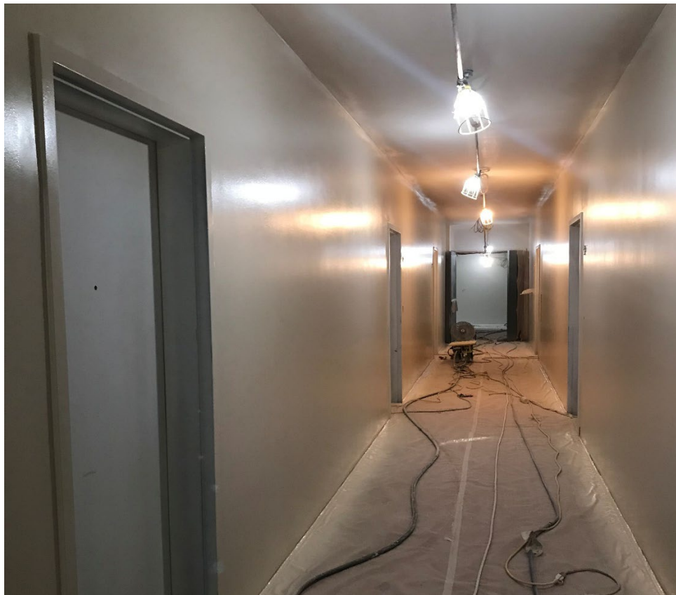
Figure 7: Texture and Paint at level 4
