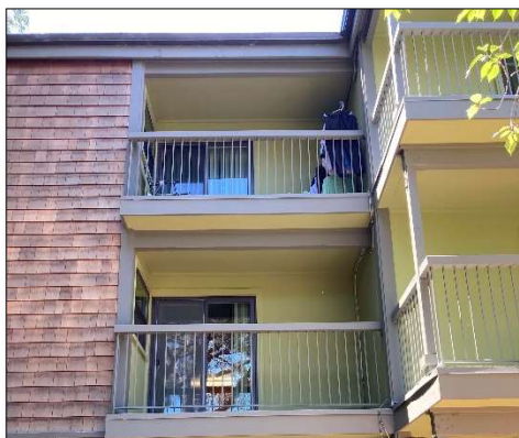
2. ABD Finished Balconies
