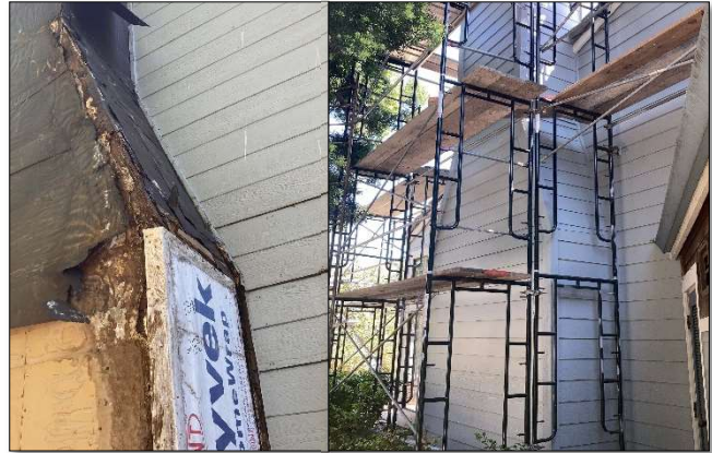
3. IP Community Room Chimney Repairs Before (left) and After (right)
