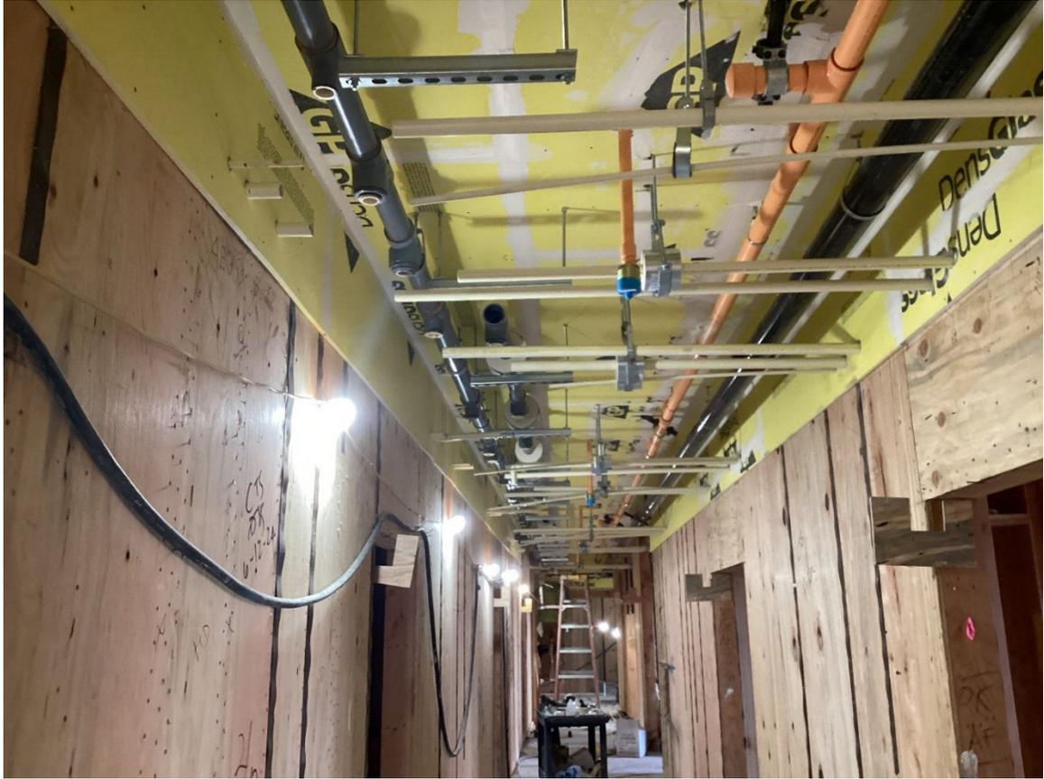
*Figure 7: View of water main installation*
