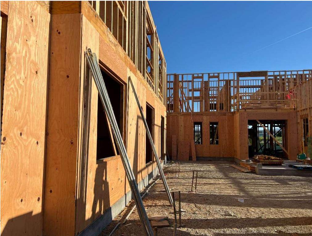
Exterior plywood sheathing installed on the eastern elevation of the first floor.
