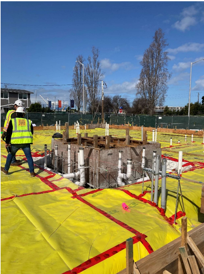
Formation and waterproofing of the elevator pit.
