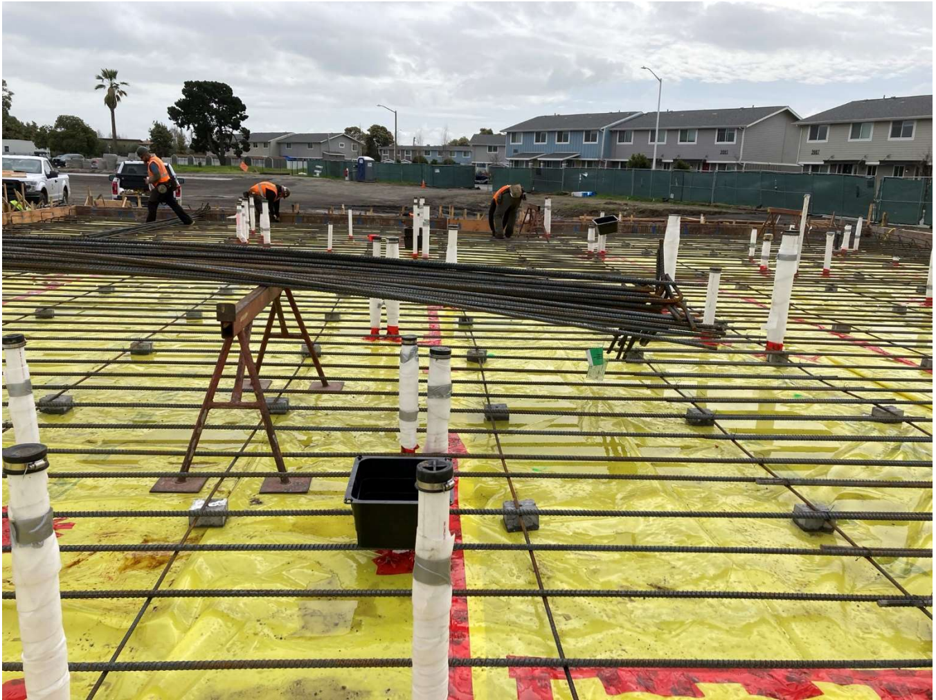
The long metal poles are rebar to reinforce the concrete for the building foundation. The white pipes are for underground plumbing.
