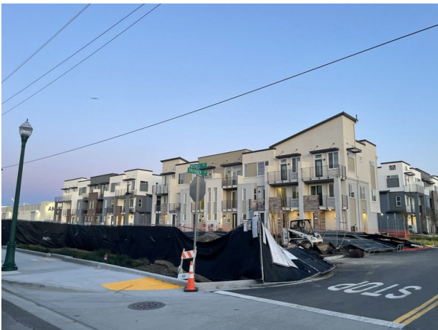
Bay 37 development further northeast
