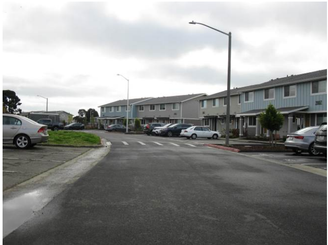
Lakehurst Circle facing south
